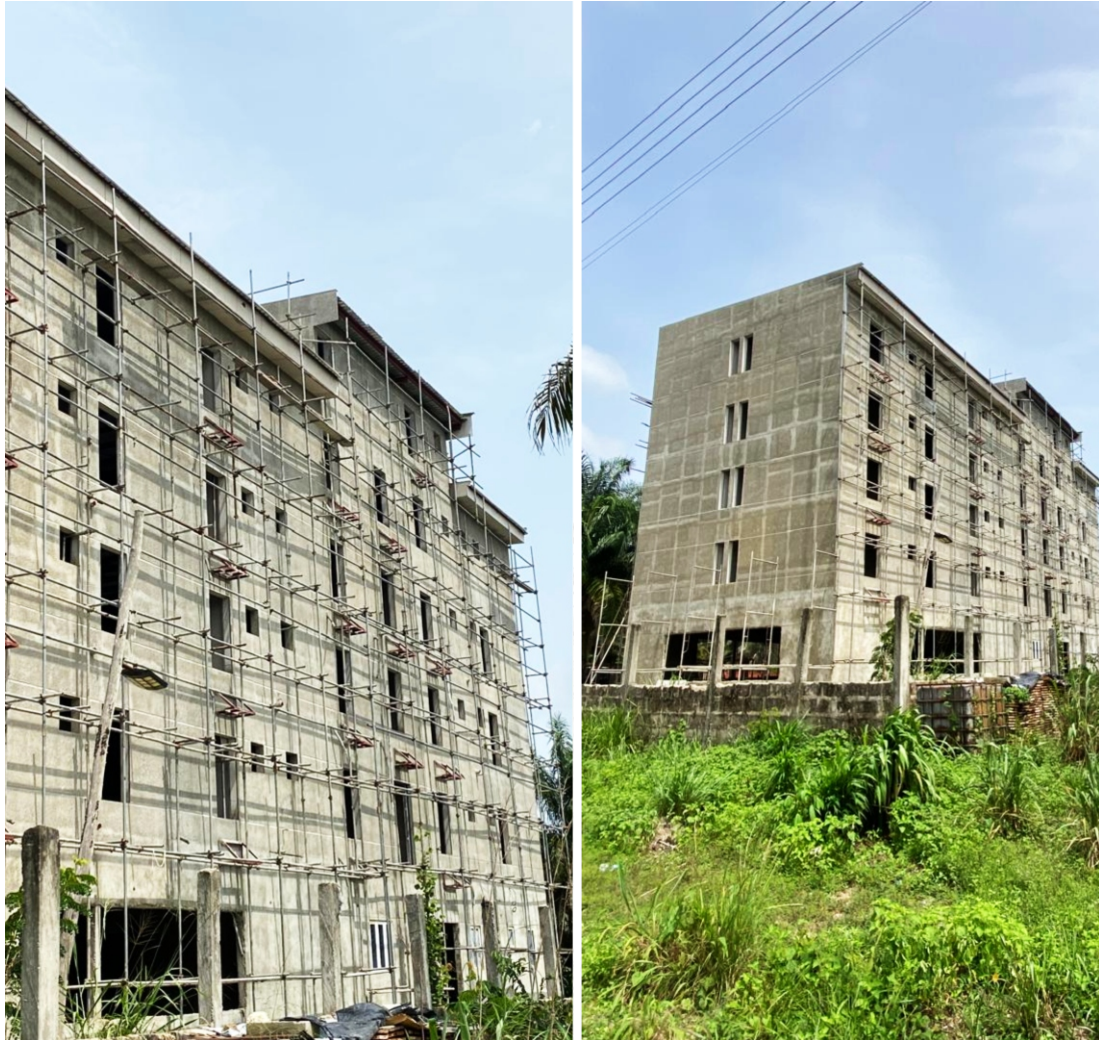
Ongoing Civil Construction of a Hundred Rooms Resort at Eku
